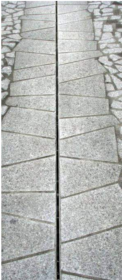
Fig. 142 Stormwater slot drain in paving Source: www.landezine.com/st-flour-pavement-by-insitu-landscape-architecture-01.jpg
