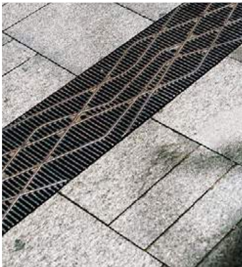
Fig. 140 Technical trench with decorative cover Source: www.landezine.com/index.php/2013/10/pitt-street-mall-by-tony-carro-architecture/
